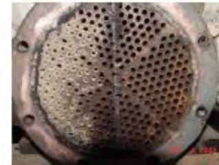
Cleaning Chemical Shell & Tube Condensor Of Chiller
